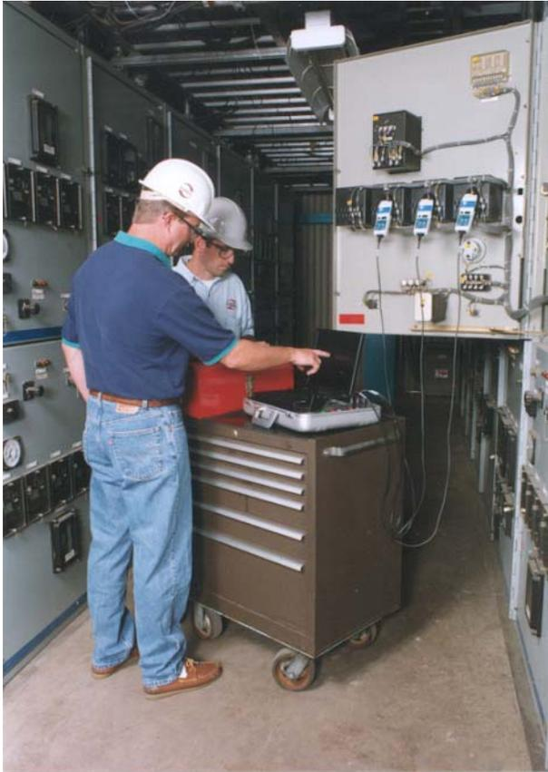
Figure 1: Using an MCEMAX to Test a High Voltage Motor
